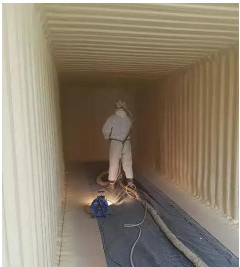
Insulation R ratings\* A 150mm thick polyurethane foam insulation layer will typically have an R-value between R-22.5 and R-42, depending on the specific type of polyurethane foam. Closed-cell spray polyurethane foam typically has an R-value of R-6.5 to R-7 per inch. Therefore, 150mm (approximately 6 inches) of closed-cell spray foam would have an R-value of roughly R-39 to R-42. Rigid foam boards, like polyisocyanurate, can also have higher R-values per inch, with some reaching R-6.5 per inches
